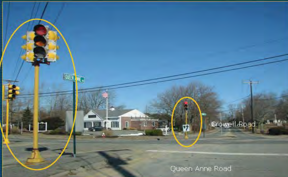
Outdated traffic signals, poor intersection geometry
